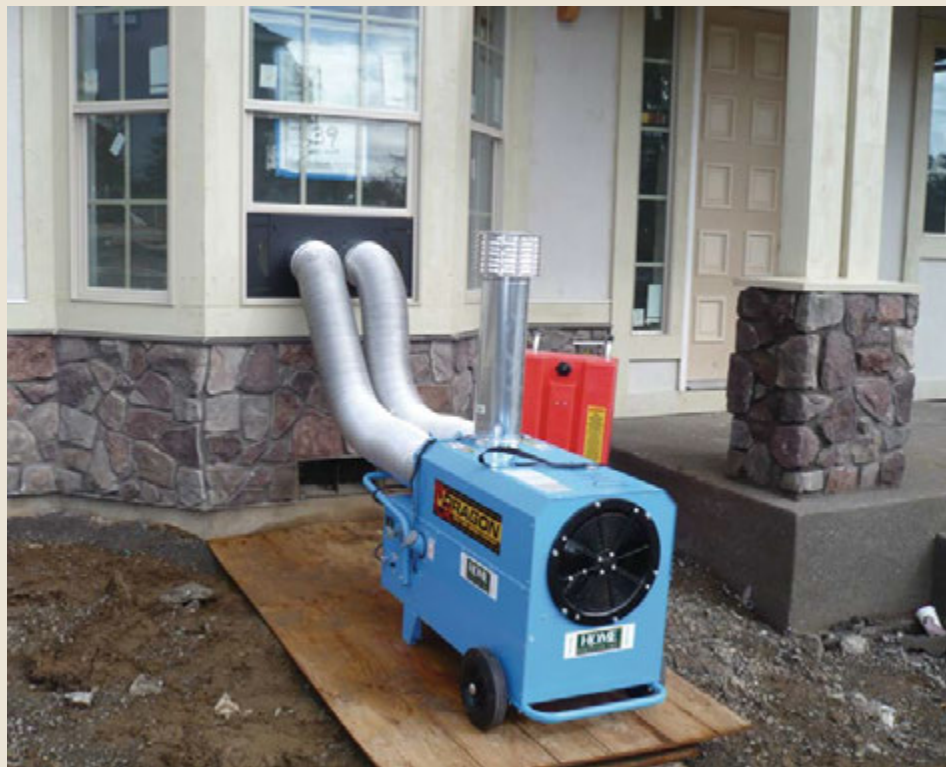
Diesel powered temporary heat when HVAC is not available.
