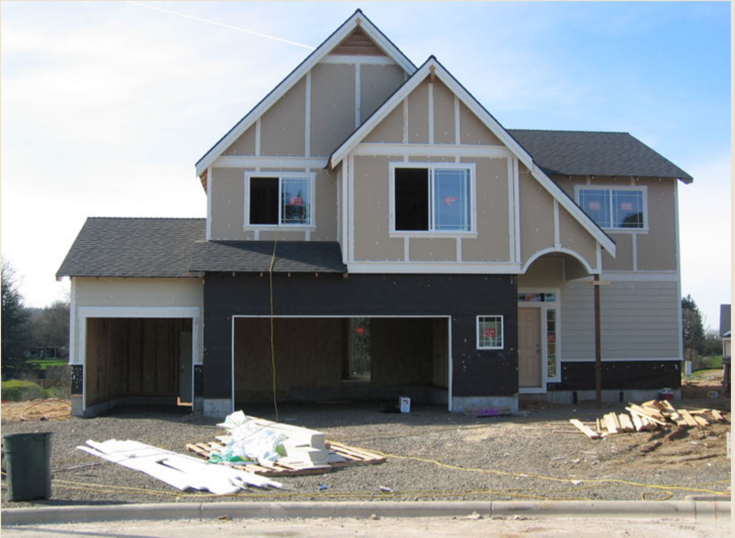
Typical stage for testing and drying of house under construction.
