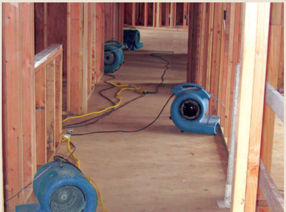
Drying equipment operating inside of house under construction.
